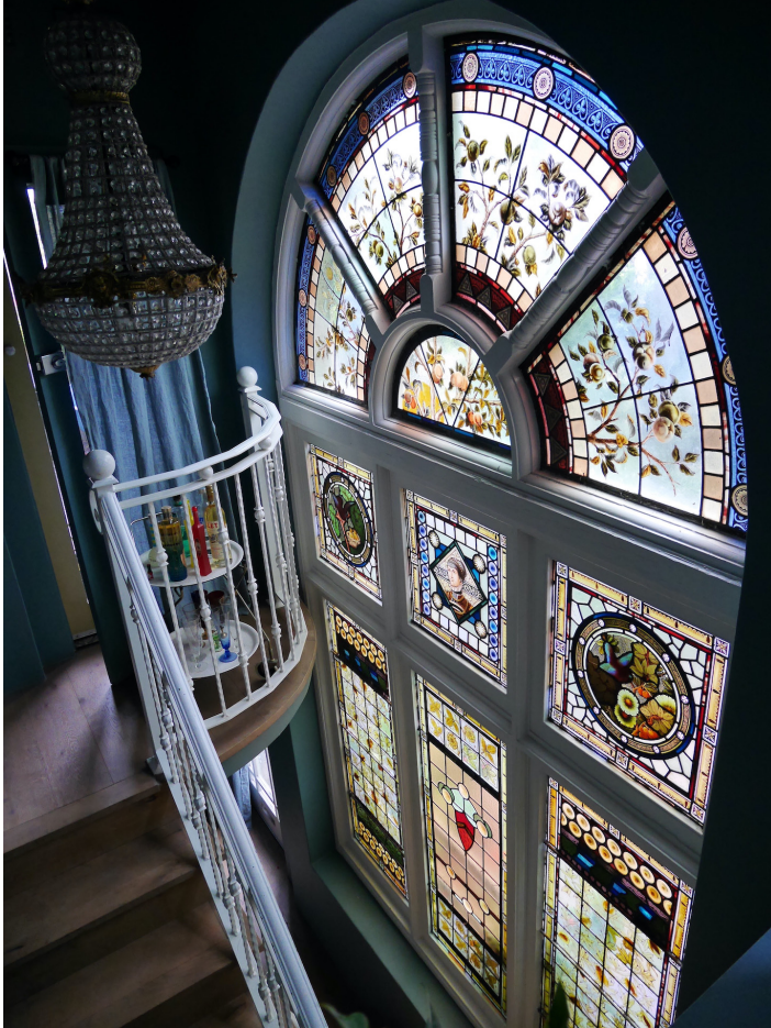
Figure 1: Lawson recycled many elements of earlier building fabrics in his landmark Beverley Hills flats (c. 1935–1936). The stunning leadlight and stained glass window in an apartment in Block 2 is believed to have come from one, or more, of the nineteenth-century mansions of Toorak that were demolished in the early 1930s. This area was originally the cafe and small shop for the complex, but has since been converted into an apartment. Personal photo supplied to the author by Heather Nette-King.
