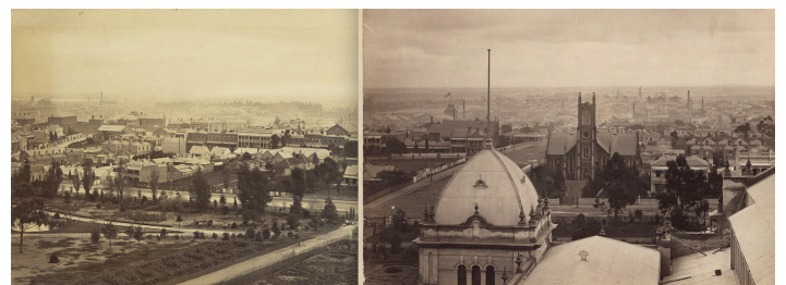
Figure 6: Composite panoramic sequence of view looking west from the roof of the Exhibition Building, Carlton Gardens, with Rathdowne Street running across the middle distance and St Andrew’s Presbyterian Church and Manse observable to the right of the dome, c. 1880 – c. 1889, State Library of Victoria, H141261 and H4570, attributed to Charles Nettleton.
