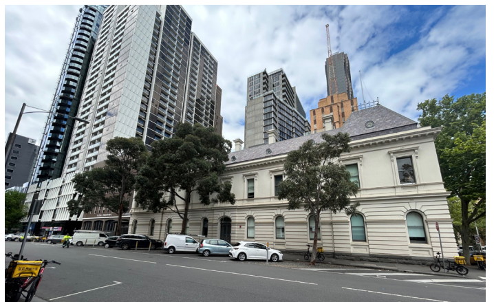
Figure 16: The two-storeyed Italian Renaissance Revival-style former police office stands on the corner of Mackenzie and Russell streets (now apartments). Next to it stands the empty, brown-brick former Victoria Police Association Building, where 45, 43 and 41 Mackenzie Street once stood. Source: Erica Cervini, 2025.
