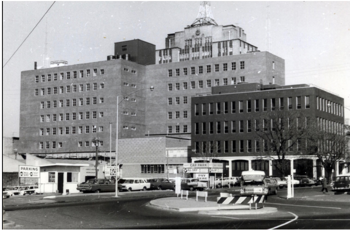
Figure 17: Mackenzie Street showing the Victoria Police Association Building in 1969. By this stage, other houses along the street had been demolished for parking bays. The Russell Street Police Headquarters, built between 1940 and 1943 (now apartments) is in the background. Source: Victoria Police Historical Society Facebook page.
