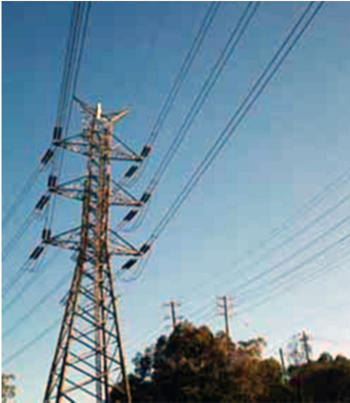
Power lines along the Merri showing the 66kV and 220kV pylons. Photograph Abigail Belfrage March 2007.
